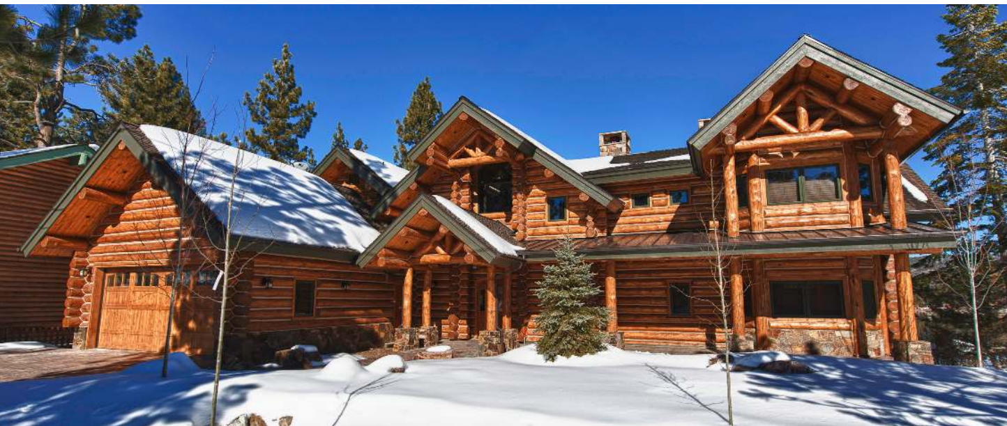
Stained with Sashco's Capture® Chestnut/Hazelnut & Cascade® Clear Coat. Photo: ©2011 Brett Christenson/Photographer
