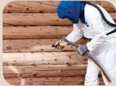
Corn Cob or Glass Blasting (Recommended method)
