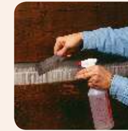
4. Lightly mist the trowel as needed.
