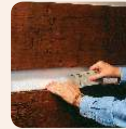
2. Tape the entire joint using polyester tape.
