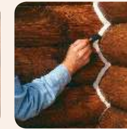
4. Tool to ensure a tight seal.
