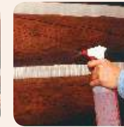
4. Lightly mist the Log Jam® as needed.
