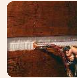
3. Gun Log Jam® over the backer material.
