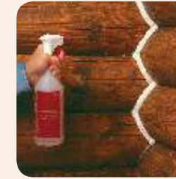
3. Lightly mist the Log Jam® as needed.
