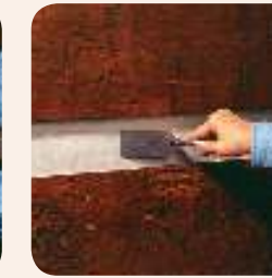
5. Tool to ensure a tight seal to the top and bottom of the chink line.
