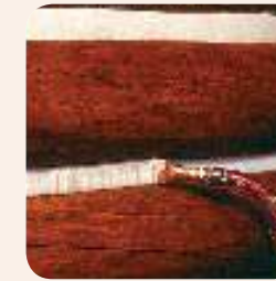
3. Gun Log Jam® over the backer rod.
