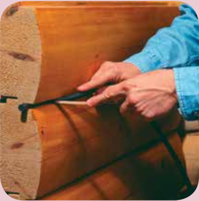
1 – Install backer rod into the caulk well of clean, stained logs.
