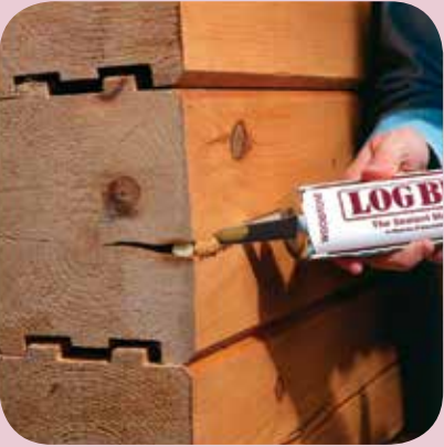
2 – Gun Log Builder over the backer rod.
