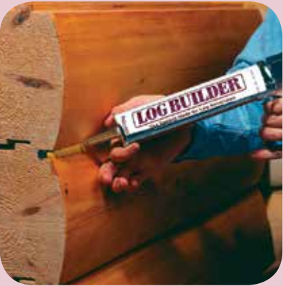
2 – Gun Log Builder over the backer rod.
