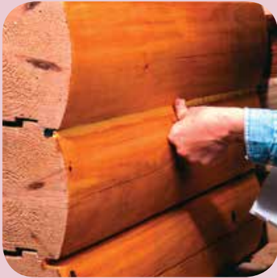
3 – Tool to ensure a tight seal to the top and bottom of the caulk line.
