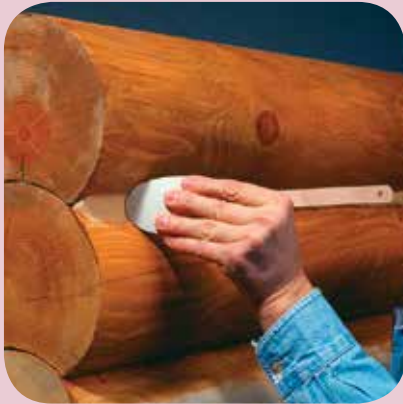
2 – Tool to ensure a tight seal to the top and bottom of the caulk line leaving at least 1/4” depth of caulk in the center of the joint.*
