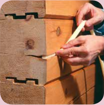
1 – Install backer rod into a clean, stained check to the appropriate depth. (See Fundamental Application Guidelines.)
