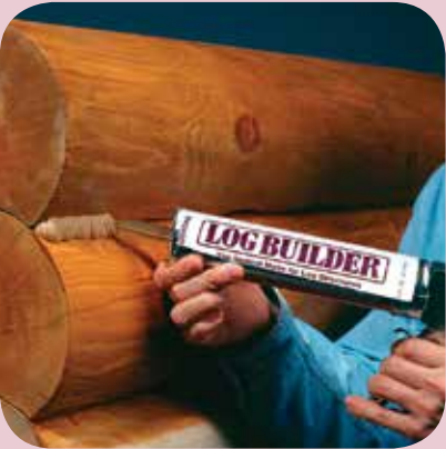
1 – Gun Log Builder into clean, stained joints.*
