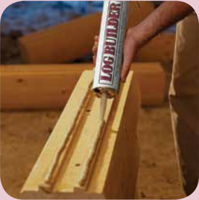
Apply bead(s) according to the log home manufacturer’s instructions. Stack the next log and repeat. Don’t allow caulk to skin over prior to stacking.
