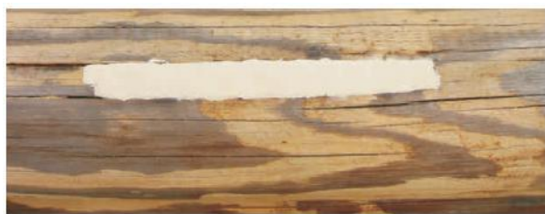
Cavity filled with E-Wood.
