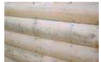
Dark colored streaks caused by metallic tannates. Oxcon solution will also remove rust stains caused by nails, screws and fasteners.
