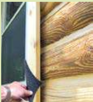
Use Log Gap Cap™ where round logs meet window and door jamb trim
