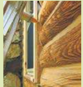
Fill the 3/8" gap between the surface of the foam and the edge of the frame with sealant
