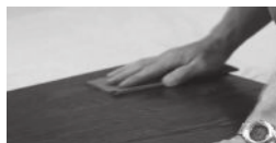
SANDING #120-#150 GRIT WITH THE GRAIN
